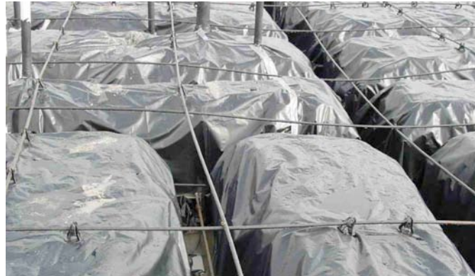
Figure 3.8-7 Example of a discontinuous rib under construction.
