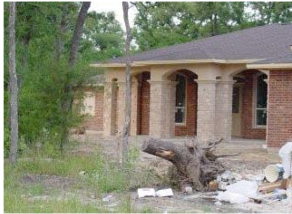
Figure 2.3.2-1 Tree stump removed from beneath the building footprint.
