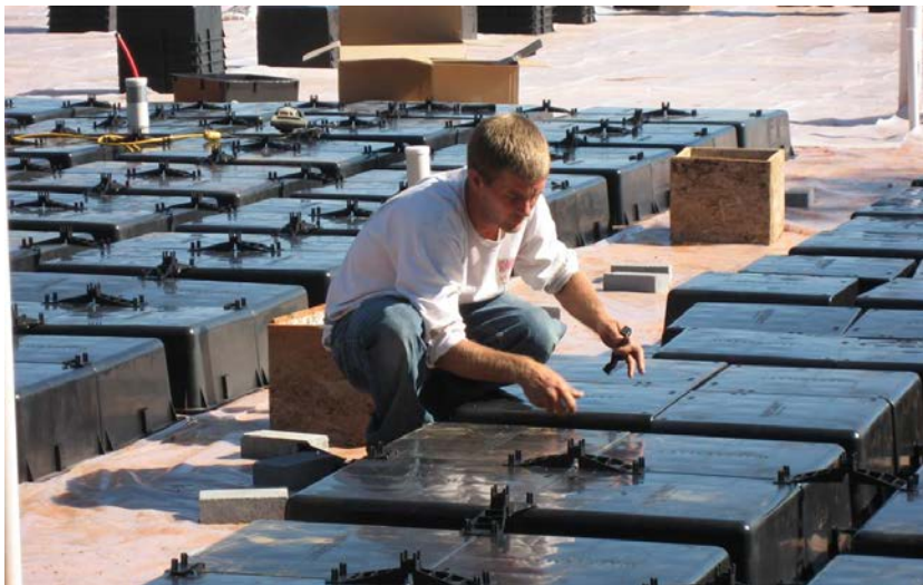
Installation of Plastic Void Forms
