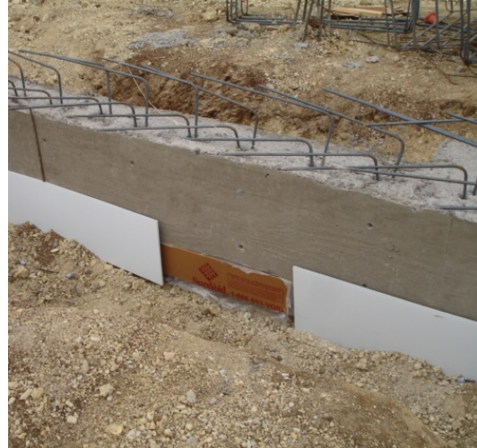
Example of high-density polypropylene (HDPP) Soil Retainers adjacent to Corrugated Paper Void Form placed under Grade Beams, designed to be vertically positioned.
