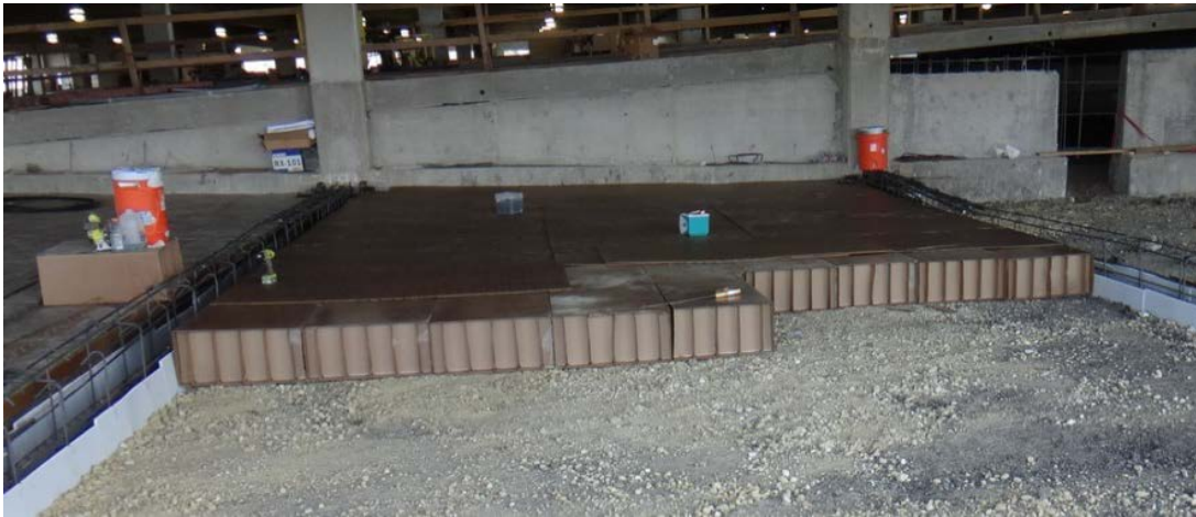
Void Forms Under Slab Area and Between Below-Ground Formed Grade Beams
