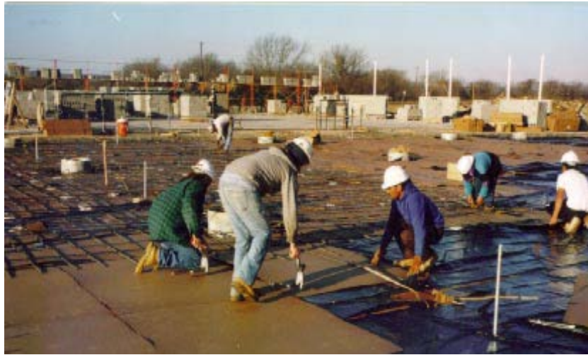
Protective fiberboard sheets being placed over Corrugated Paper Void Forms
