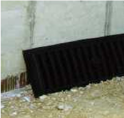
Example of a high-density polyethylene (HDPE) Soil Retainer manufactured of materials that are not adversely affected by moisture, designed to be positioned at an angle.
