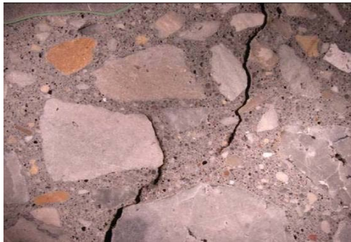
Figure 2.17.8 Typical plastic shrinkage cracking
