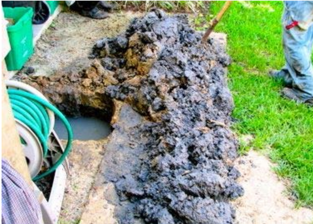
Figure 2.12.1 Excavation at Foundation Edge Showing High Water Table
