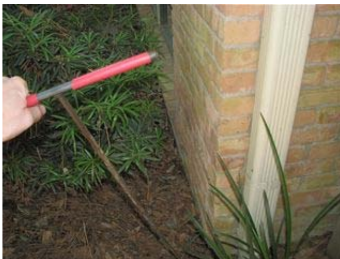
Figure 2.8.1 Ground Probing at a perimeter grade beam
