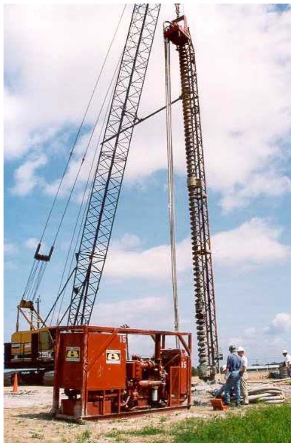
Figure 1. ACIP pile rig
