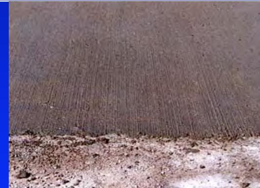
The final poured concrete that is poured on top of JointDrain in order to repair 2 faulty concrete joints.
