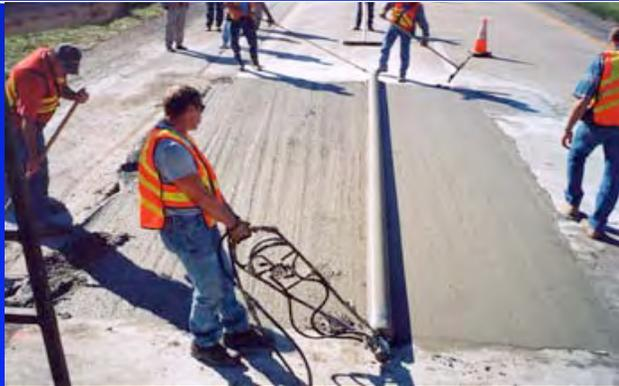
After a couple of passes of the screed, the concrete is ready for finishing touches.
