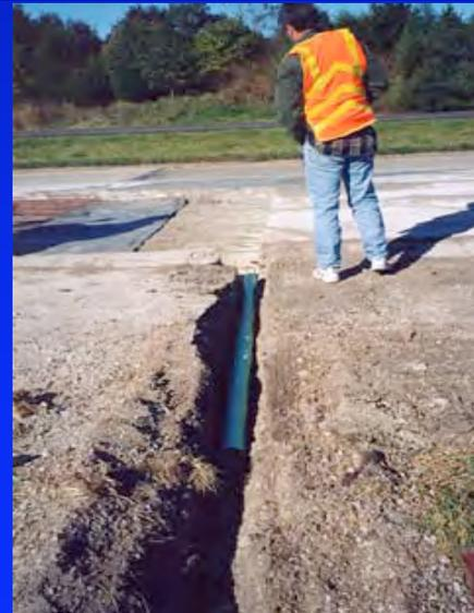
**A Perforated PVC Pipe is placed as a drainage outlet at the end of the 25' section.**
