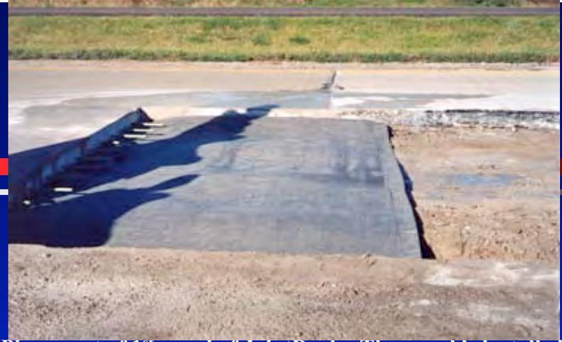
**Placement of 1<sup>st</sup> panel of JointDrain. The panel is installed under the dowel bars with the main drainage path going toward the drainage trench.**
