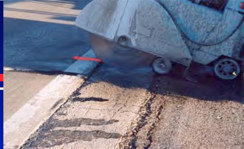
**Cutting out a 25' section of concrete
