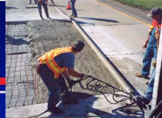
Screed is used to smooth and flatten the poured concrete.
