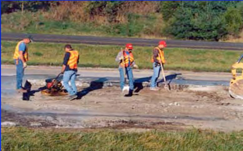
**Clearing debris to prepare subgrade**
