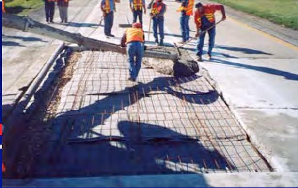
Ready-mix concrete is poured directly on JointDrain panels.
