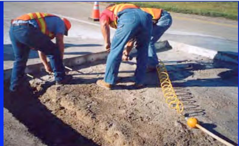
**Placement of dowel rods**
