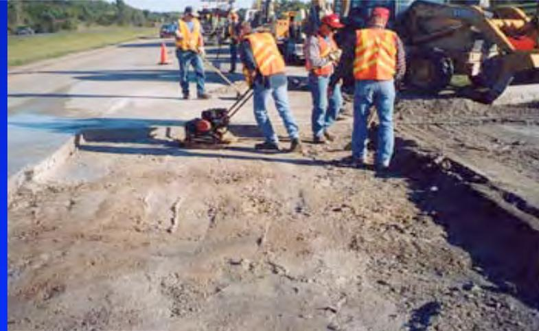
**Compacting subgrade in preparation for
