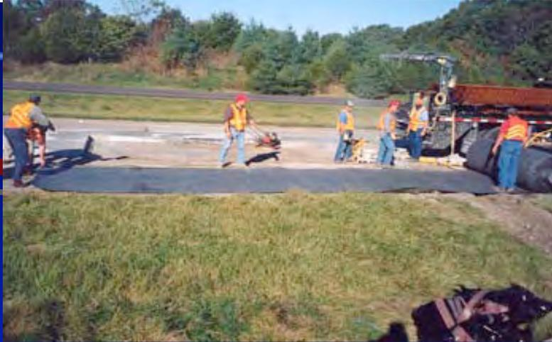
**Rolling out material to cut a 12'x24' JointDrain panel. Rolls come in 6.7' and 12' widths and lengths of 200 ft.**
