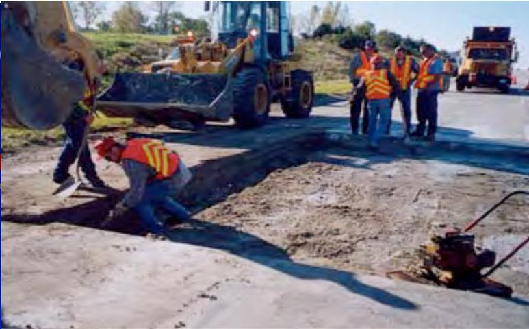
**A drainage trench must be dug at the edge of the road to collect moisture that drains through the JointDrain.**
