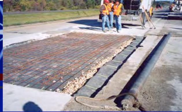
After last panel of JointDrain is placed, metal mesh is placed. Metal mesh is rested on dow bars, and on top of JointDrain panel.
