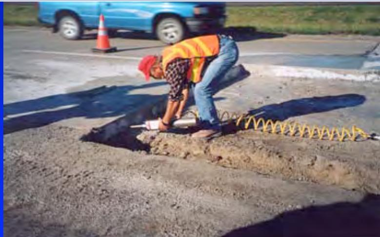
**Applying epoxy into dowel holes before placement of dowel rods**
