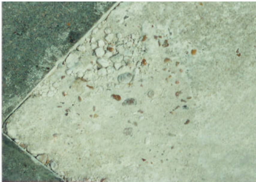
Figure 5. A Close-up of the Concrete Patch Located to the South of the Food Mart (The concrete is cracking and spalling, and aggregates are falling apart.)
