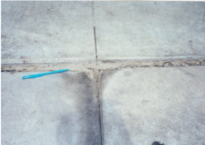
Figure 4. A View of the Faulting (Stepping) Joint Crack Located to the East of the Northern Driveway
