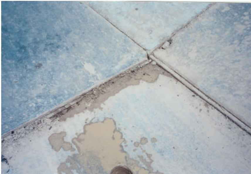
Figure 3. A View of the Expansion Joint with Missing Sealant and Deteriorated Wooden Insert Located to the Southeast of the RV Service Island (Subgrade fines mixing with water were pumped out when heavy trucks passed by.)
