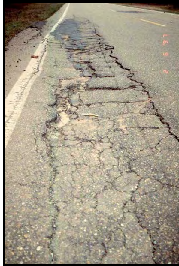
Base Failure
