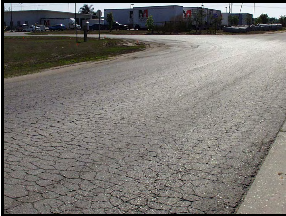
Alligator Cracking
