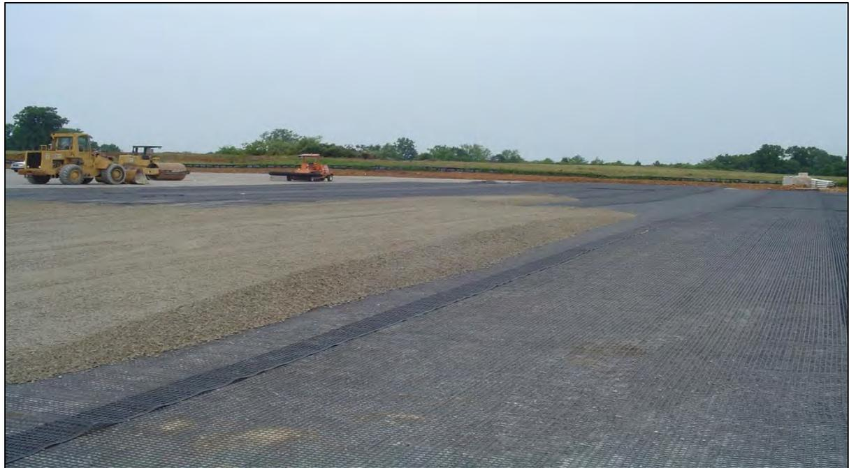
SF11 was produced in 17' x 200' rolls to increase installation efficiency
