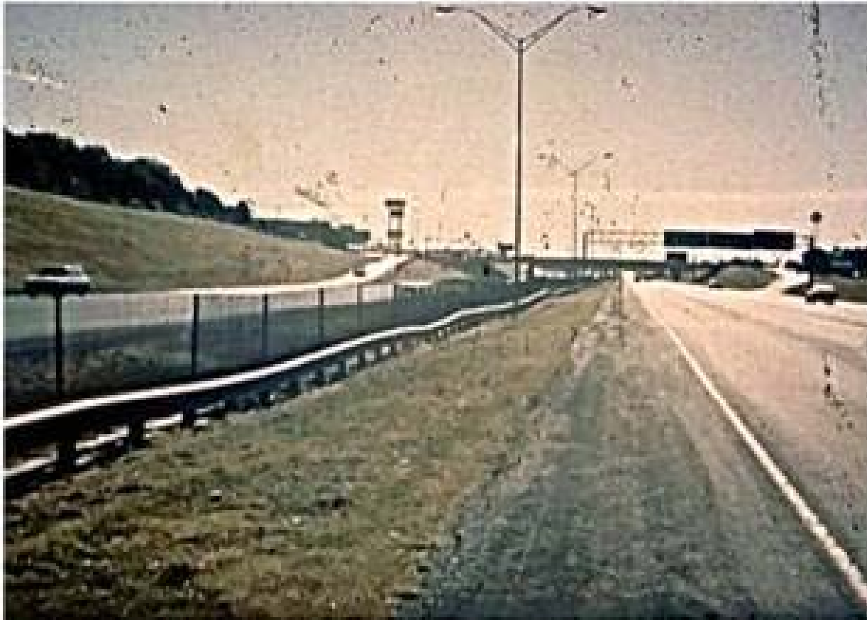
Guardrail between pavement lanes on expansive clay subgrade IH37, San Antonio, Texas (c. 1974)
