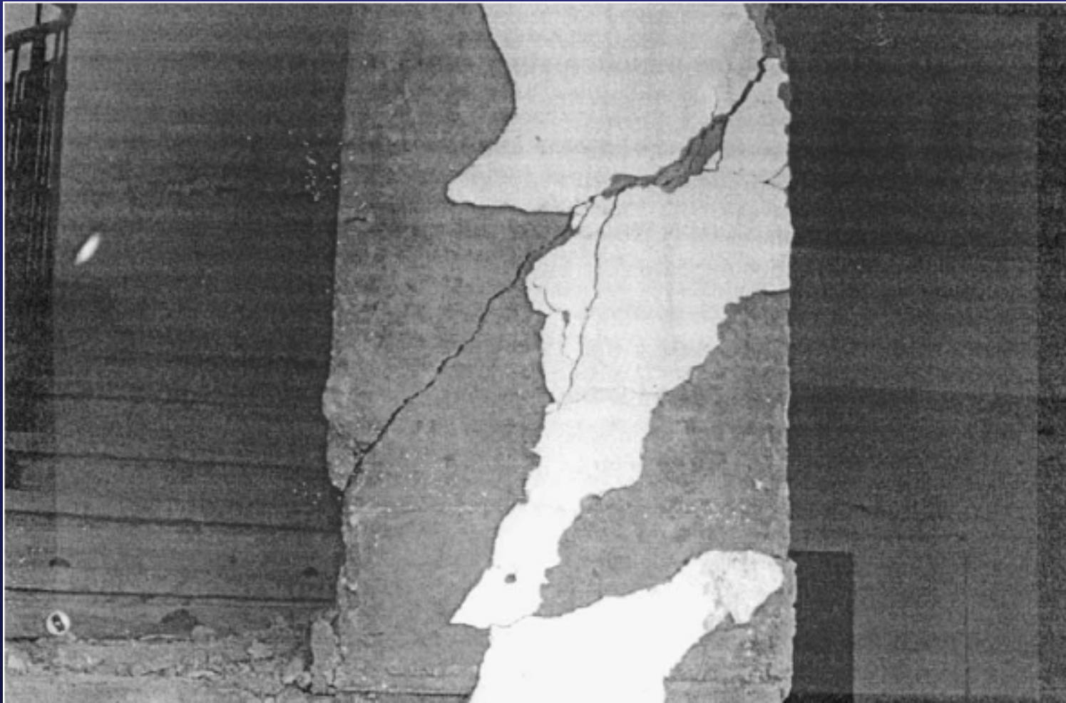
Severe damage to a reinforced concrete columns due to differential heave, in Saudi Arabia (Al-Shamrani and Dhowian, 2003)
