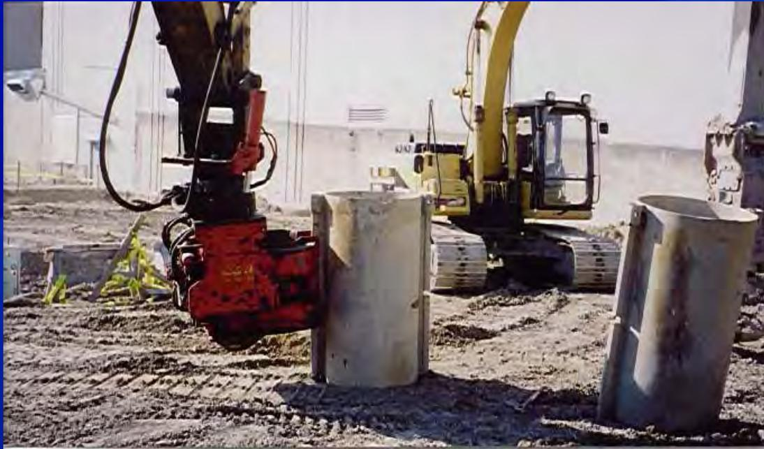
**Temporary casing used to stabilize caving soils**
