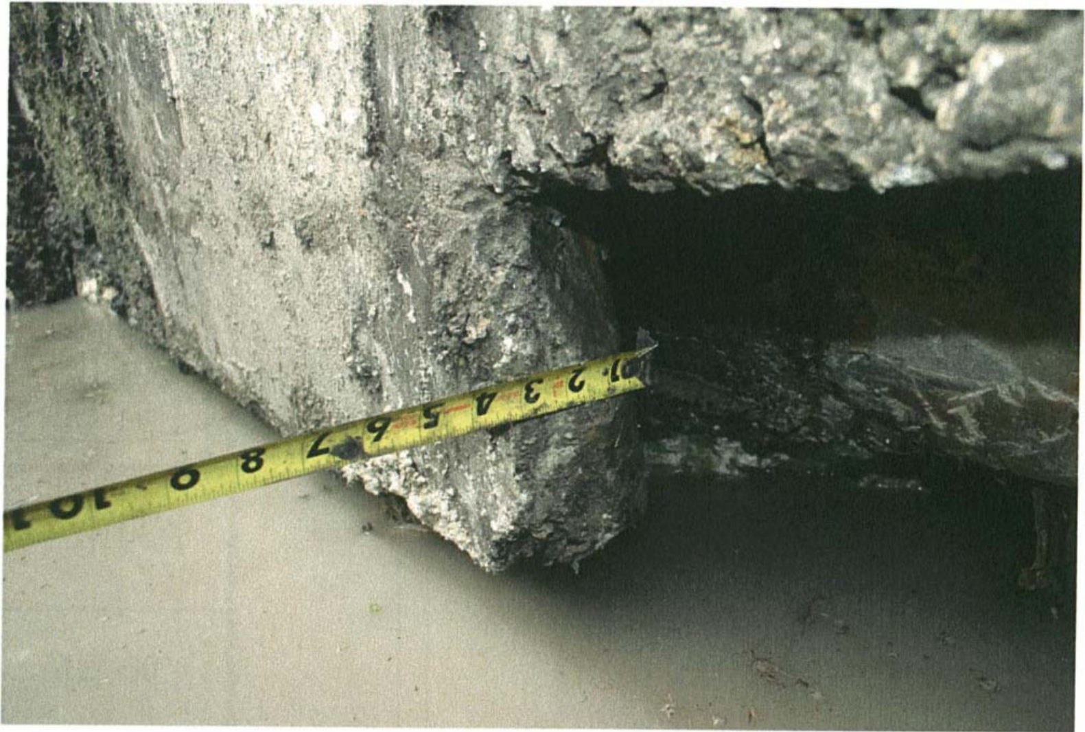
Test Pit #1: Two carton forms. Inside collapsed. Outside left 3.5" concrete in contact with clay.
