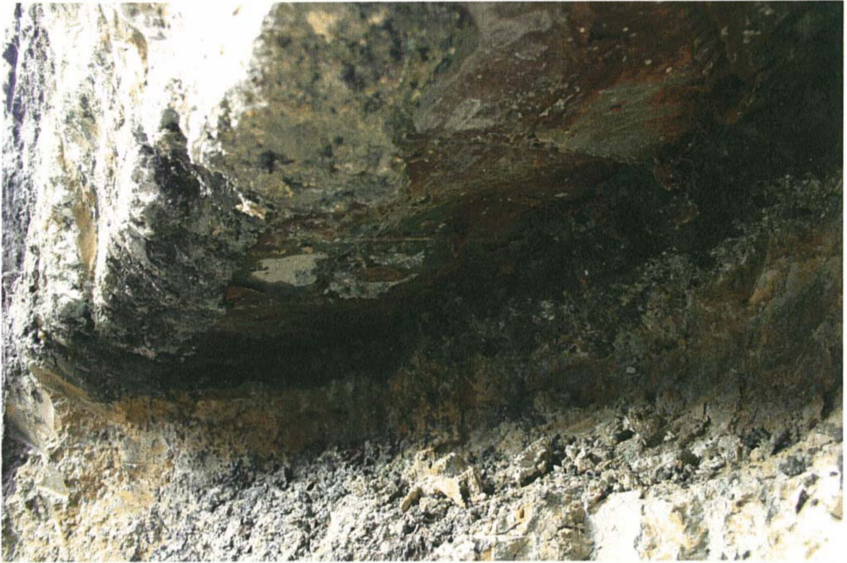
Test Pit #3, no void, carton form collapsed.
