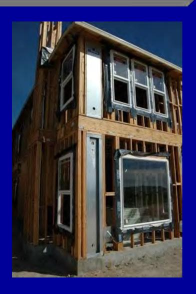
Is there enough room for the panel and the cripple studs supporting the header?
