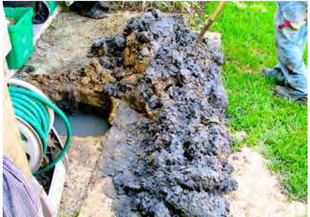
Test pit excavation
