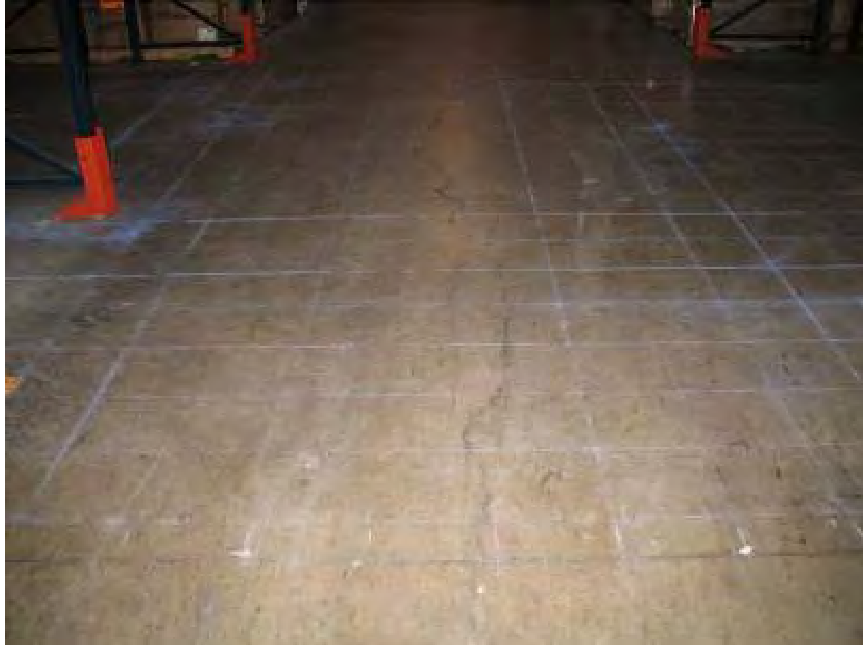
Grid layout for detailed crack mapping area
